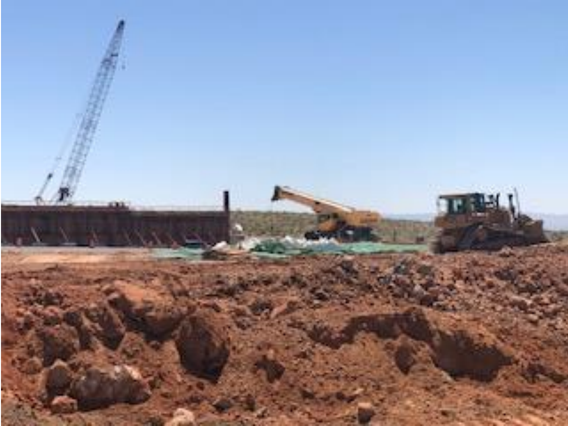
Road Construction of future overpass at SR-9
